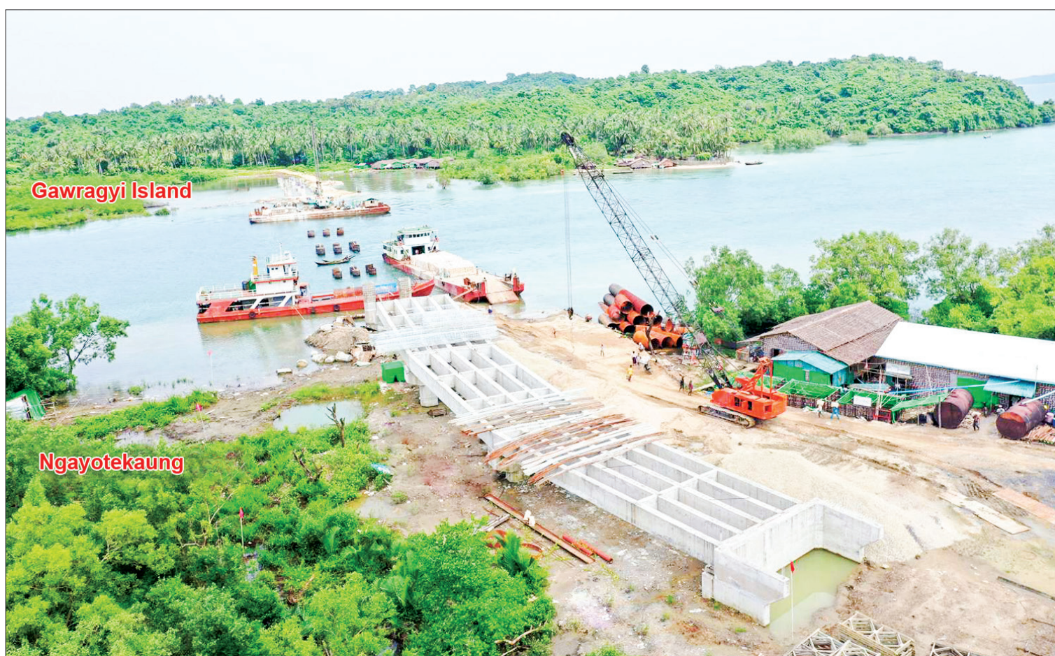
An aerial view of the project site. PHOTO: SOE MYINT AUNG
