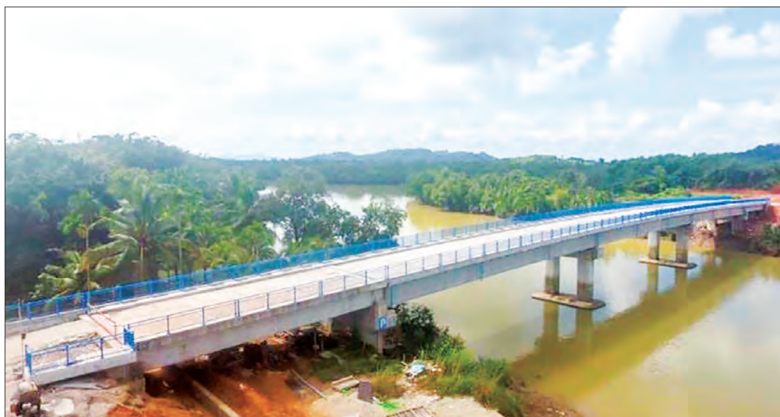
An aerial view of the Yezin Chaung Bridge. PHOTO: SOE MYINT AUNG
