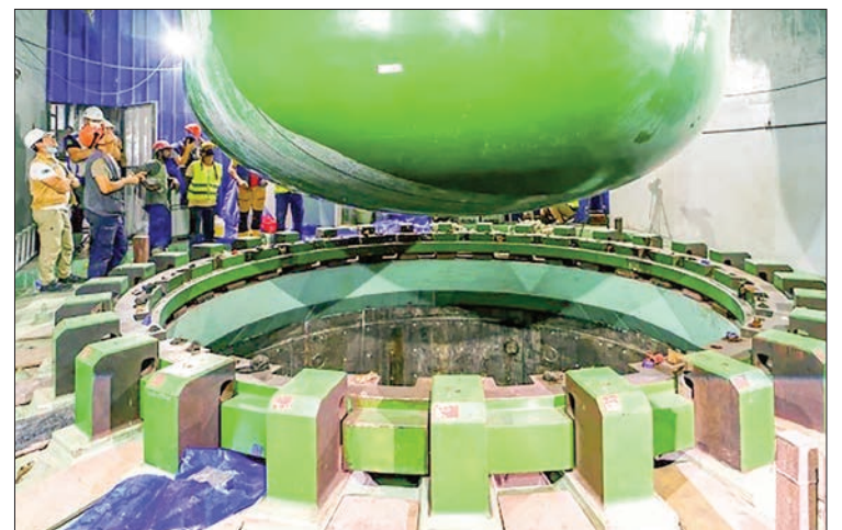
Rooppur 1’s reactor pressure vessel is manoeuvred into position. PHOTO: ROSATOM/ANI
