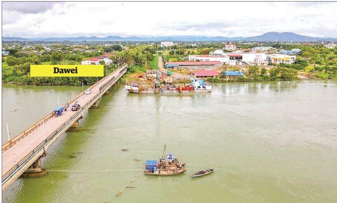
Kamyawkin bridge construction site. PHOTO: SOE MYINT AUNG
