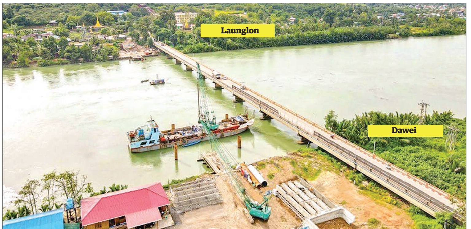
Kamyawkin bridge construction site. PHOTO: SOE MYINT AUNG
