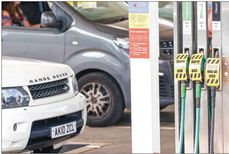
"Out of Use" pumps are pictured at a Tesco petrol station in Camberley, west of London on 26 September 2021. PHOTO: ADRIAN DENNIS / AFP
