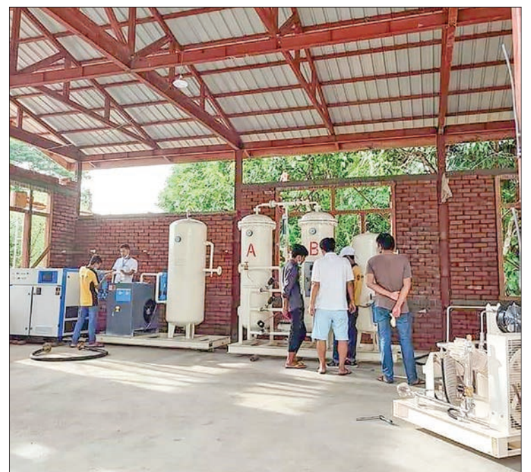
The construction project is being carried out by the Mawlaik district committee on control and emergency response to COVID-19 in cooperation with residents and departmental staff. PHOTO: MAW LAIK IPRD.
