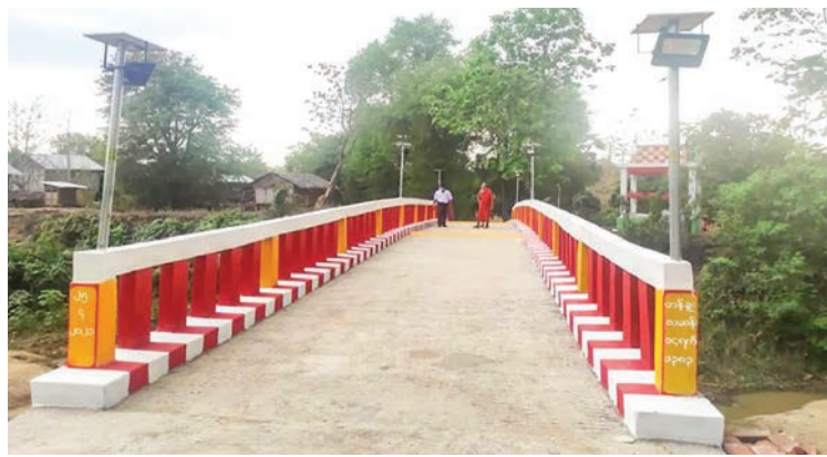
A concrete bridge repair work reaches completion.
