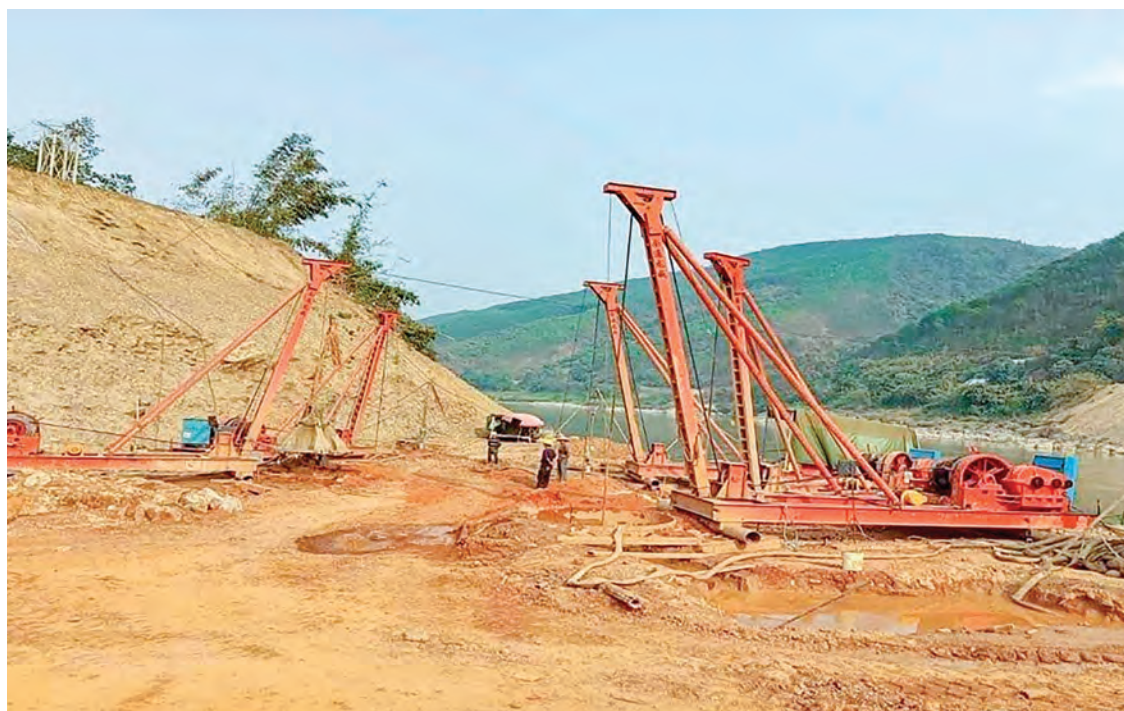
Foundation work is underway.
