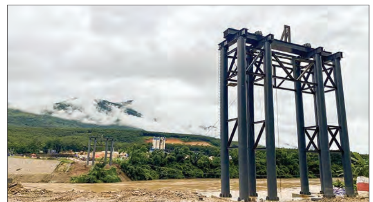
Construction site of the Kunlong Bridge.
