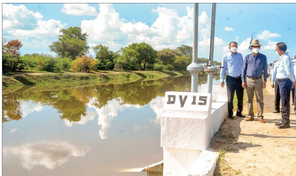
MoALI Union Minister U Tin Htut Oo and party inspects the irrigation system of Kintar Reservoir and Kintar Diversion Weir in Myittha Township in Mandalay Region on 1 September 2021.
