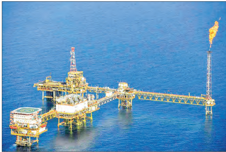
This undated handout picture provided by PETRONAS shows their Sabah gas platform off the coast of Sabah, on northern Borneo island. PHOTO: PETRONAS MALAYSIA / AFP/FILE
