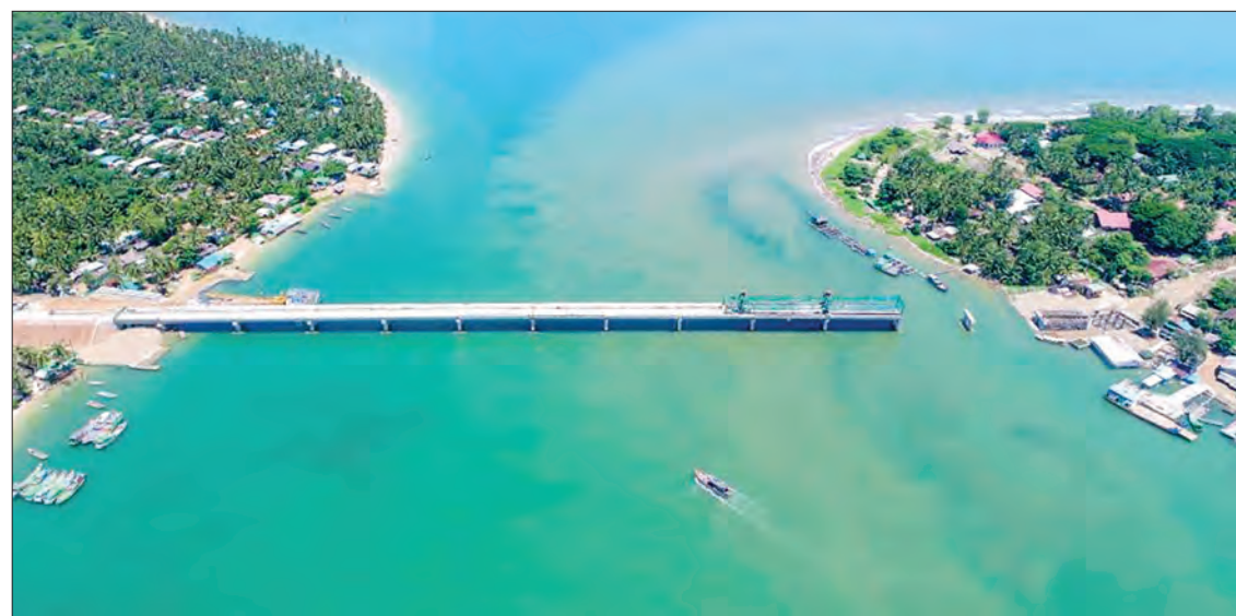
The construction site of the Gwachaung Bridge. PHOTO: SOE MYINT AUNG
