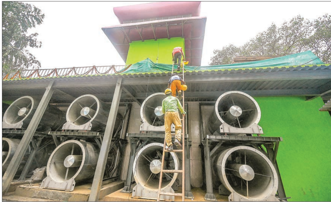
Workers climb a ladder at the 25-metre (82-foot) high smog tower, built to purify the air during pollution season, in New Delhi on 23 August 2021. PHOTO: MONEY SHARMA / AFP
