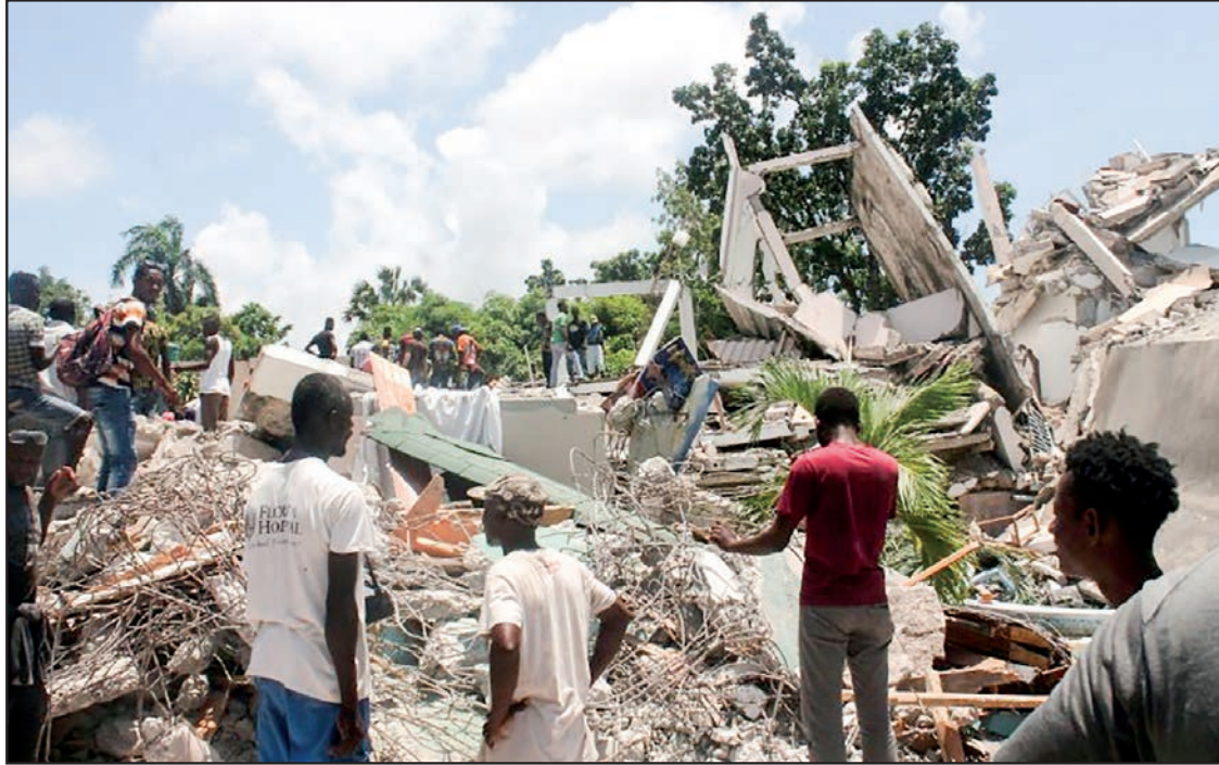
Rescuers are racing against the clock to find survivors in the rubble of buildings destroyed by the quake, including the remains of the Manguier Hotel in Les Cayes. PHOTO: AFP
