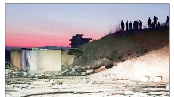
The site of the overnight fuel tank explosion in Lebanon's northern region of Akkar - the remains of the tank are visible to the left. PHOTO: AFP
