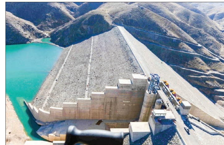
This photograph taken on December 2, 2015, shows a general view of the Salma hydroelectric dam in Chishti Sharif, in the eastern part of Herat Province. PHOTO: AREF KARIMI/AFP/FILE
