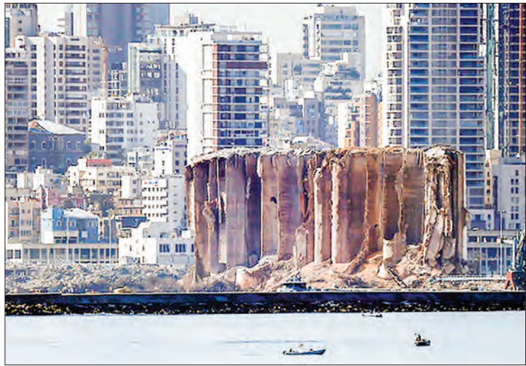
Destroyed silos at Beirut's port following the 4 August massive chemical explosion. PHOTO: AFP
