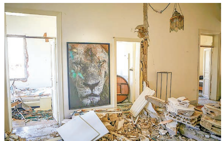
A view shows the damage inside an apartment in the neighbourhood of Gemmayze on 5 August 2020, a day after a blast in a warehouse in the port of the Lebanese capital sowed devastation across entire city neighbourhoods, killing more than 100 people, wounding thousands and plunging Lebanon deeper into crisis. PHOTO: PATRICK BAZ / AFP
