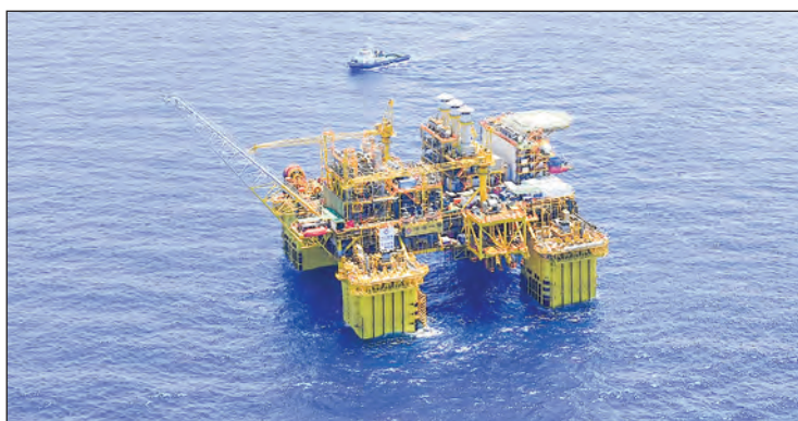
Deep Sea No 1, a semi-submersible oil production and storage facility, is located in the waters off South China’s Hainan province. PHOTO: XINHUA
