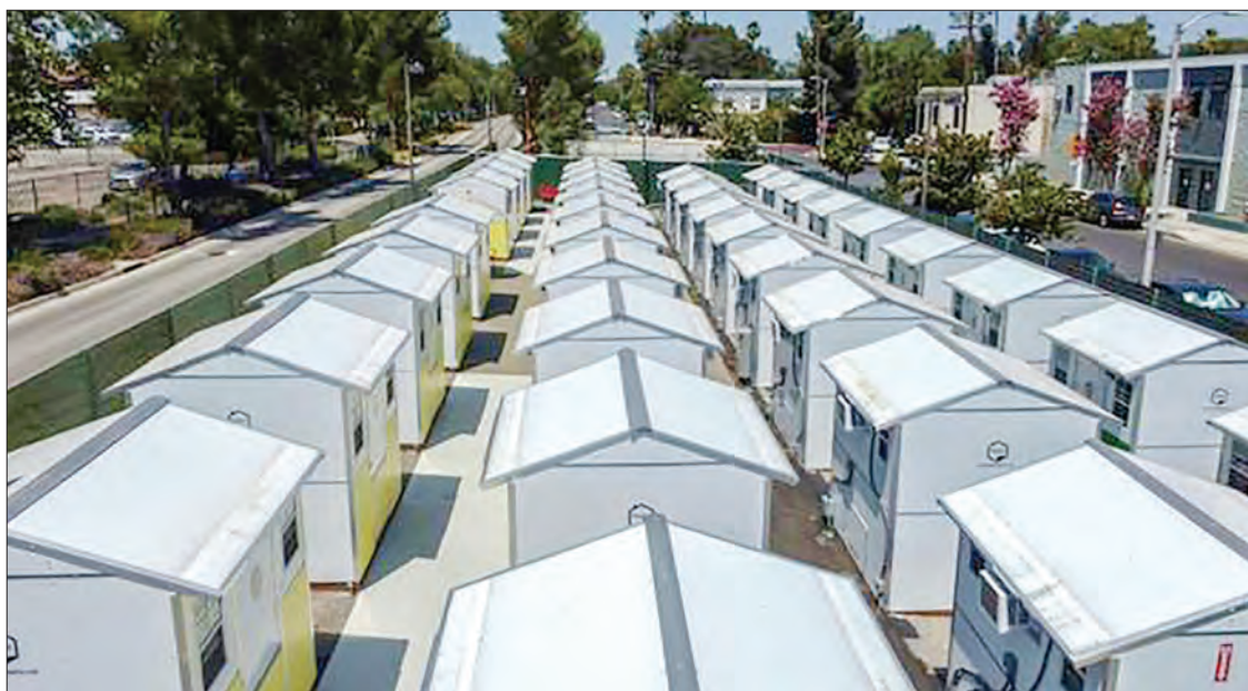
Los Angeles has established several "tiny home villages", including this one in the Tarzana neighbourhood, to help the homeless. PHOTO: AFP
