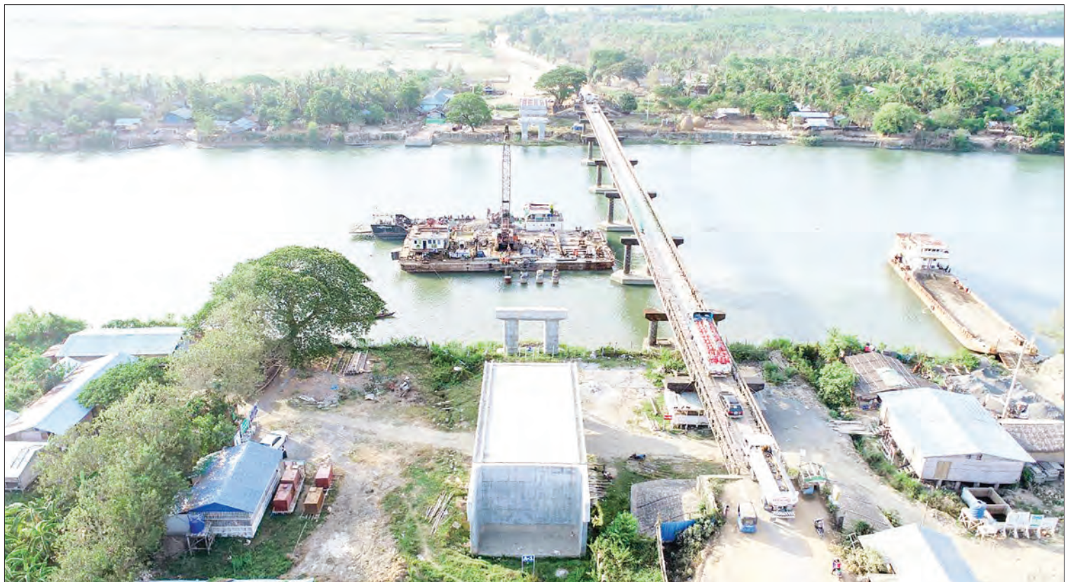
Myaung Bway bridge construction site in Rakhine State.
