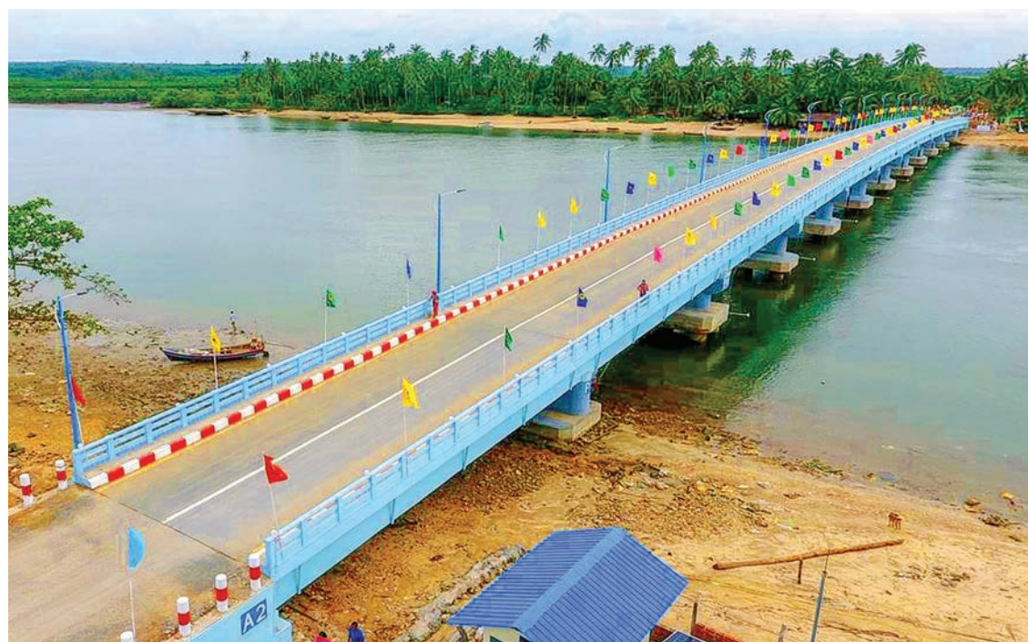
An aerial view of the Shwethoungyan Bridge on the Chaungtha-Shwethoung Road.
