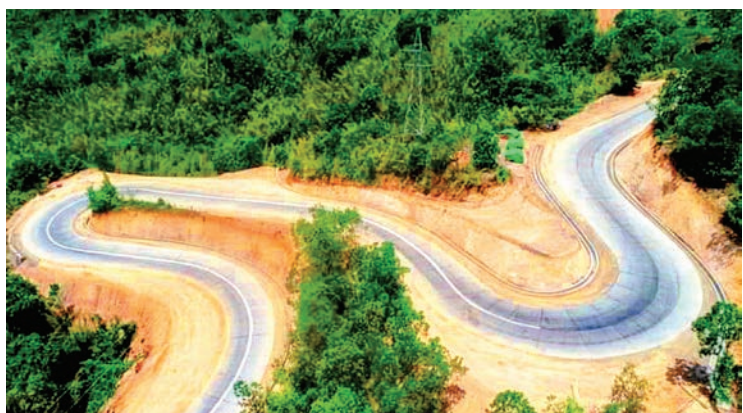
The Pathein-Yangon Highway emerges as a development instance of Ayeyawady.
