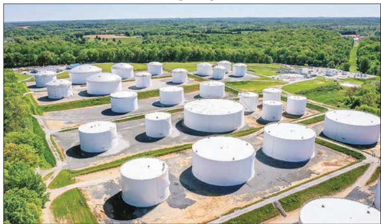
Fuel holding tanks are seen at Colonial Pipeline's Dorsey Junction Station, which was shut down by a cyberattack that disrupted gas supply for the eastern US for days, highlighting the growing threat hackers pose to infrastructure. PHOTO: AFP/FILE
