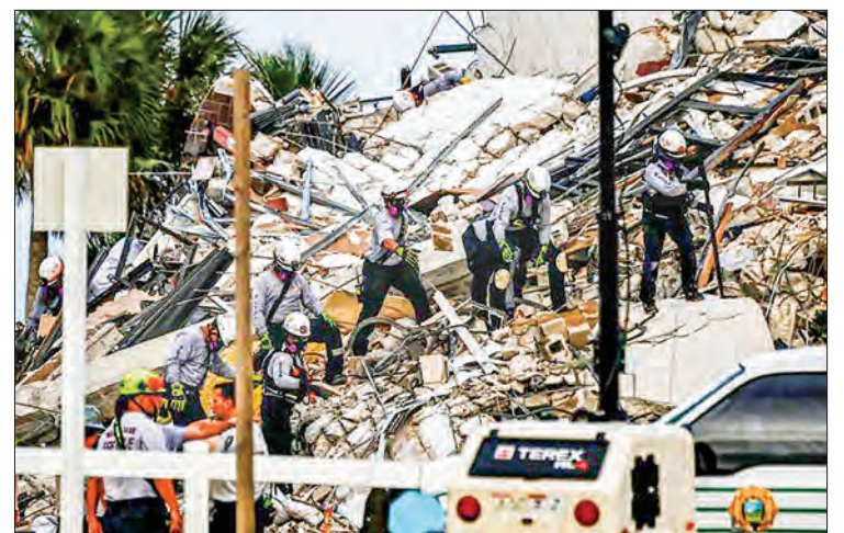
US Search and Rescue personnel work at a partial collapse building in Surfside, Miami Beach. PHOTO: AFP
