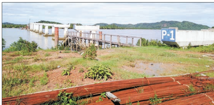
The concrete Min Than-Maung Hlaw bridge is 2,100 feet long, 33 feet wide and is of 26 feet of water clearance height.
