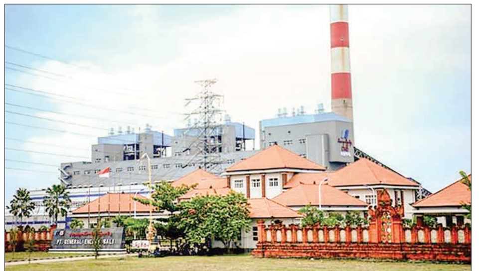
The Celukan Bawang 2 power plant in Singaraja on Indonesia's resort island of Bali is seen in October 2020. PHOTO: AFP/FILE
