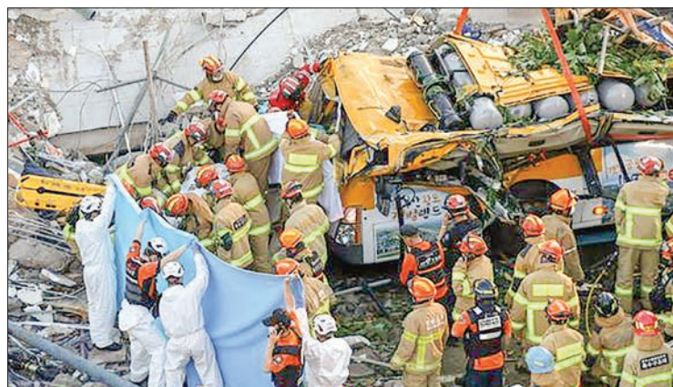
South Korean rescue workers search for survivors in the debris of a collapsed building in Gwangju. PHOTO: YONHAP/AFP
