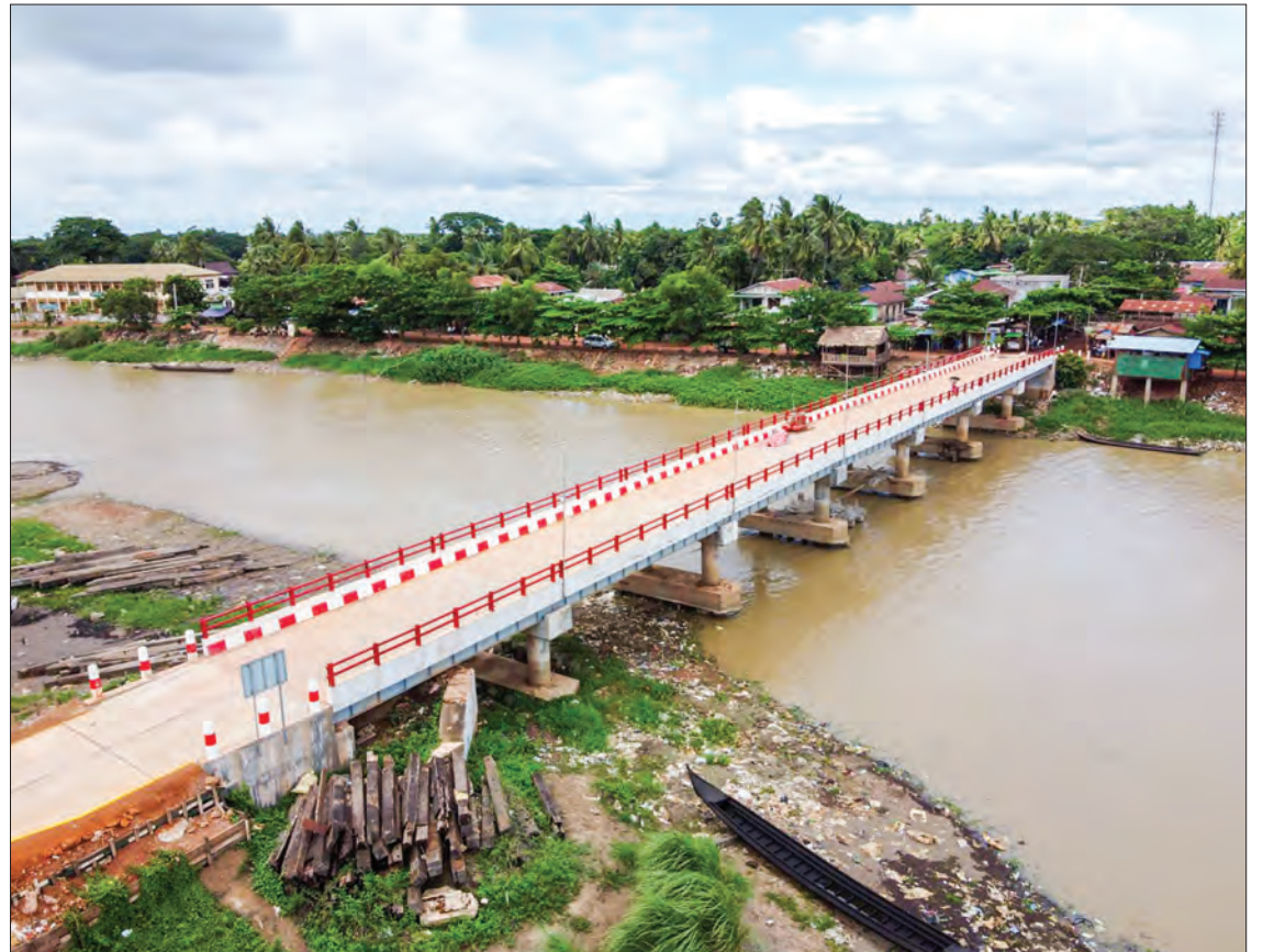
The concrete bridge, with a bored pile foundation, has a load capacity of 30 tonnes. The bridge is 260 feet long and 18 feet wide. The bridge clearance is 9 feet.
