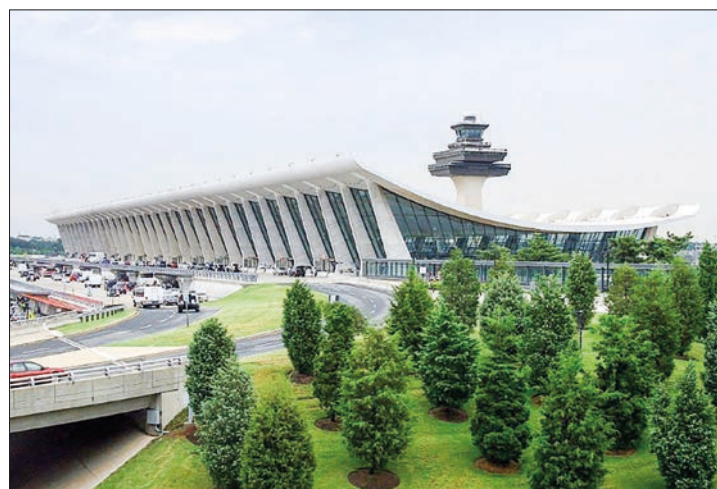
The Colonial Pipeline serves millions of customers on the East Coast, including Washington Dulles International Airport. PHOTO: AFP
