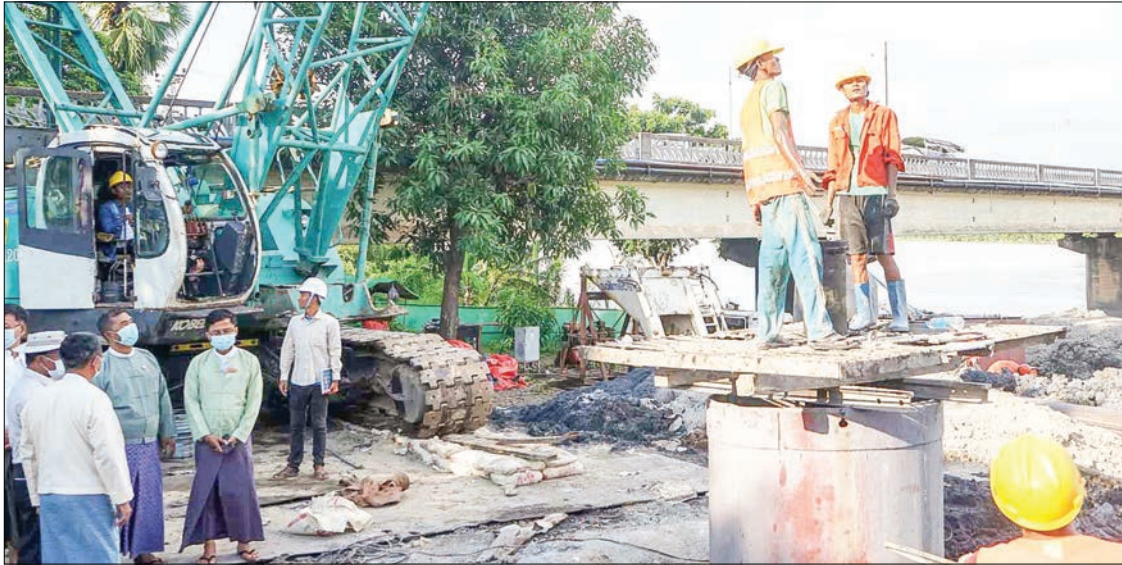
The Kamyawkin Bridge construction work in progress.
