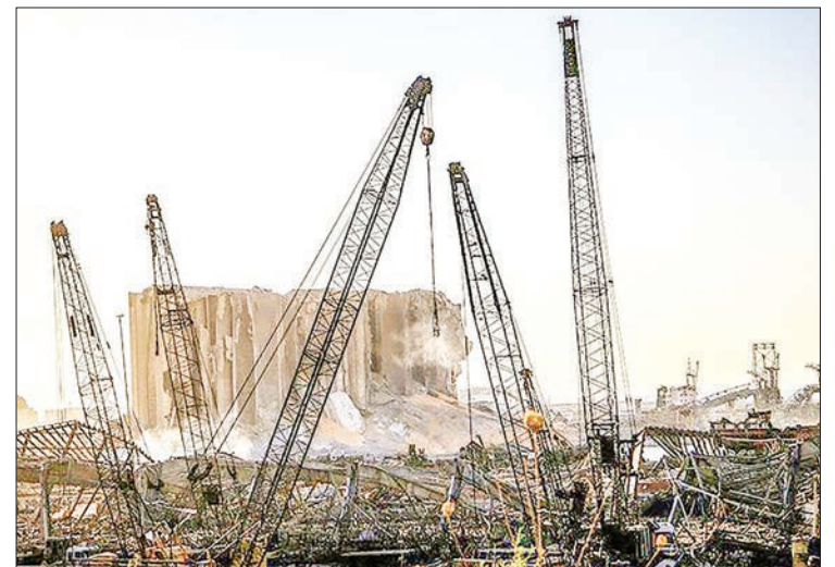
The August 4 explosion of hundreds of tons of ill-stored fertilizers devastated the docks and large swathes of the capital, killing more than 200 people. PHOTO: AFP
