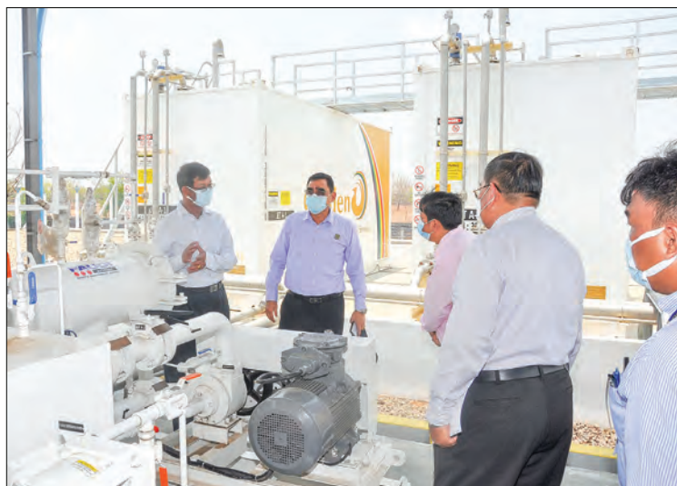
The MoTC deputy minister is inspecting the upgrading works of Bagan-NyaungU airport yesterday.
