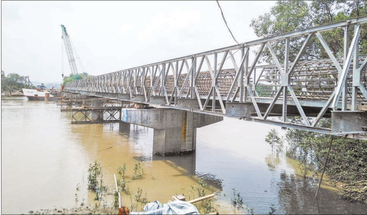
The bridge is 900 feet long and 22 feet wide, with 13 feet 9 inches’ traffic lane.
