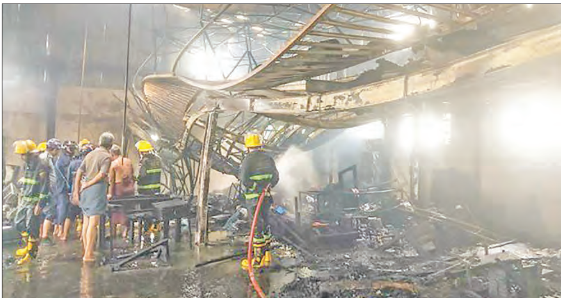
The Yoma Water Treatment Plant was ravaged by a fire yesterday.
