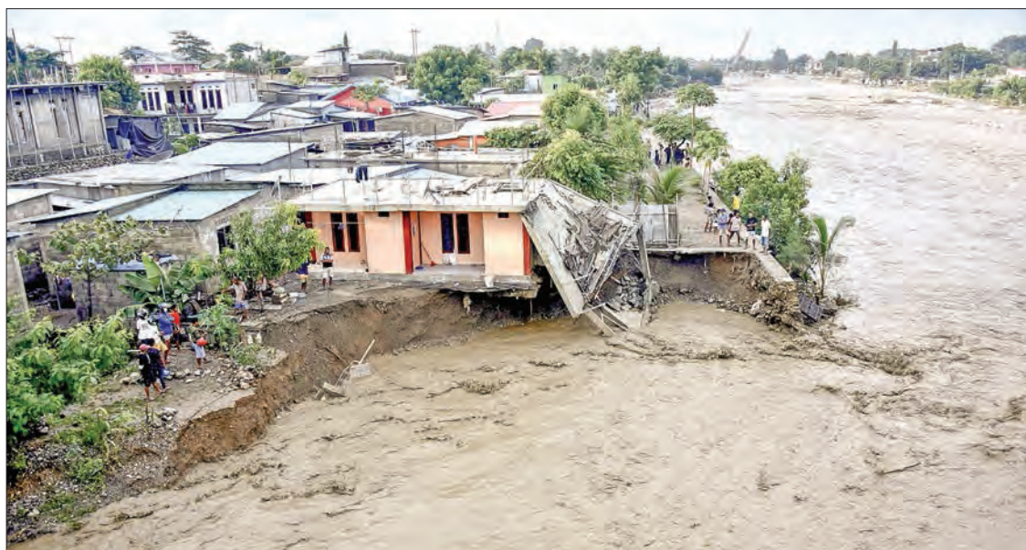
Residents stand along the water's edge by damaged homes after heavy rains and strong winds lashed East Timor's capital Dili overnight causing extensive flooding on 4 April 2021. PHOTO: AFP
