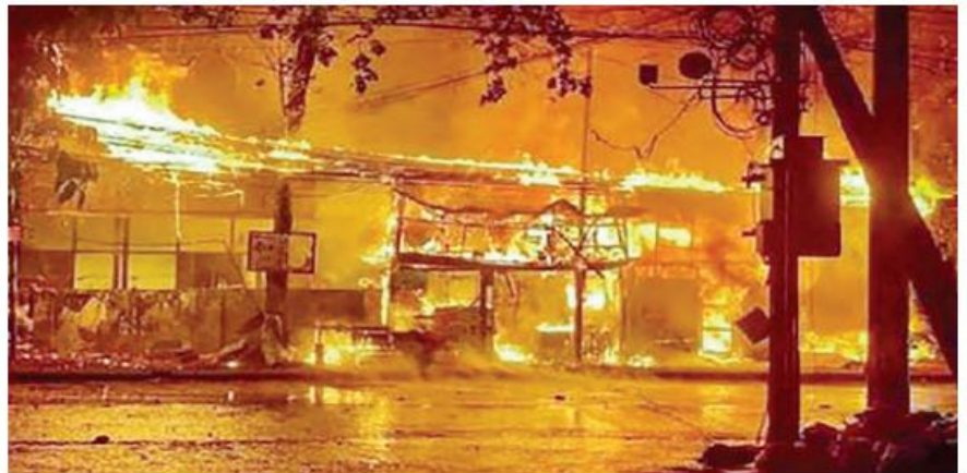
A municipal building attached to ward administration committee office seen under fire after an arson attack by violent people.
