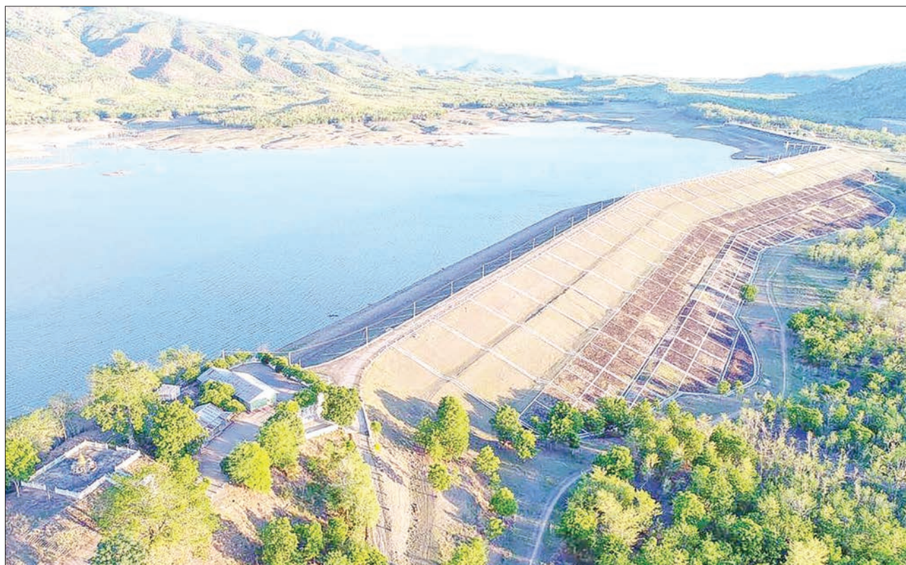
The Yinchay dam supplied the irrigation water from 1 February to 15 February to grow 150 acres of summer sesame in two farmlands, while Manchaung dam will distribute the water from 15 February to 28 February to the 15 farmlands from five village-tracts along the dam area to grow 1,000 acres of summer sesame
