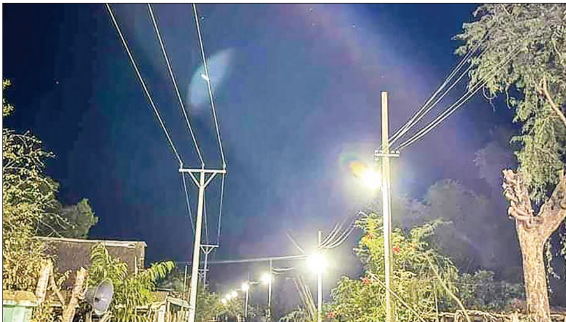
Recently about 43 villages have already access to the electricity under the NEP project.
