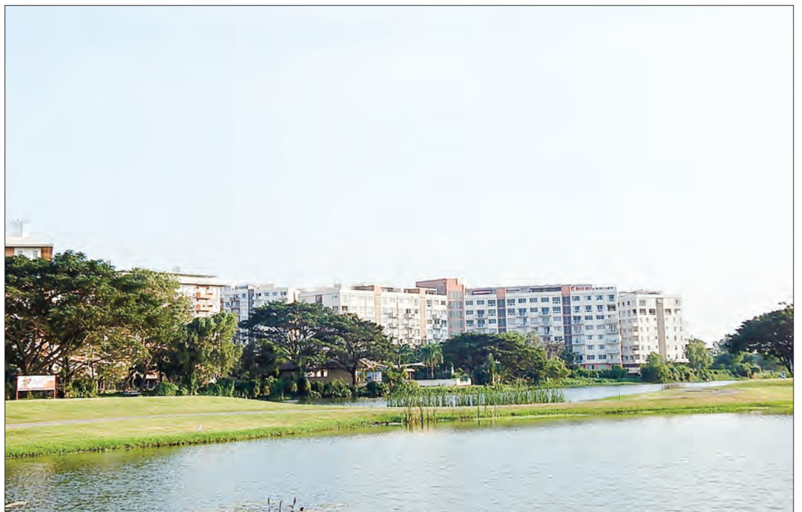
Picture shows the condominium in Thanlyin Township, Yangon Region. PHOTO: SOE MYINT AUNG
