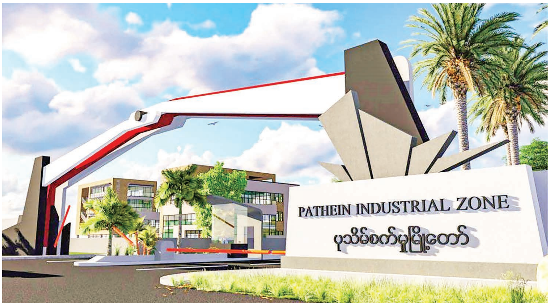
The Pathein Industrial City (PIC) project is being implemented on 6,700 acres of land in Pathein, with an investment of US$500 million. PHOTO: PICMYANMAR.COM
