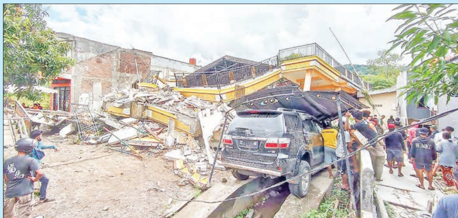
People work at the site of a collapsed building in Mamuju. MAWARDI/AFP
