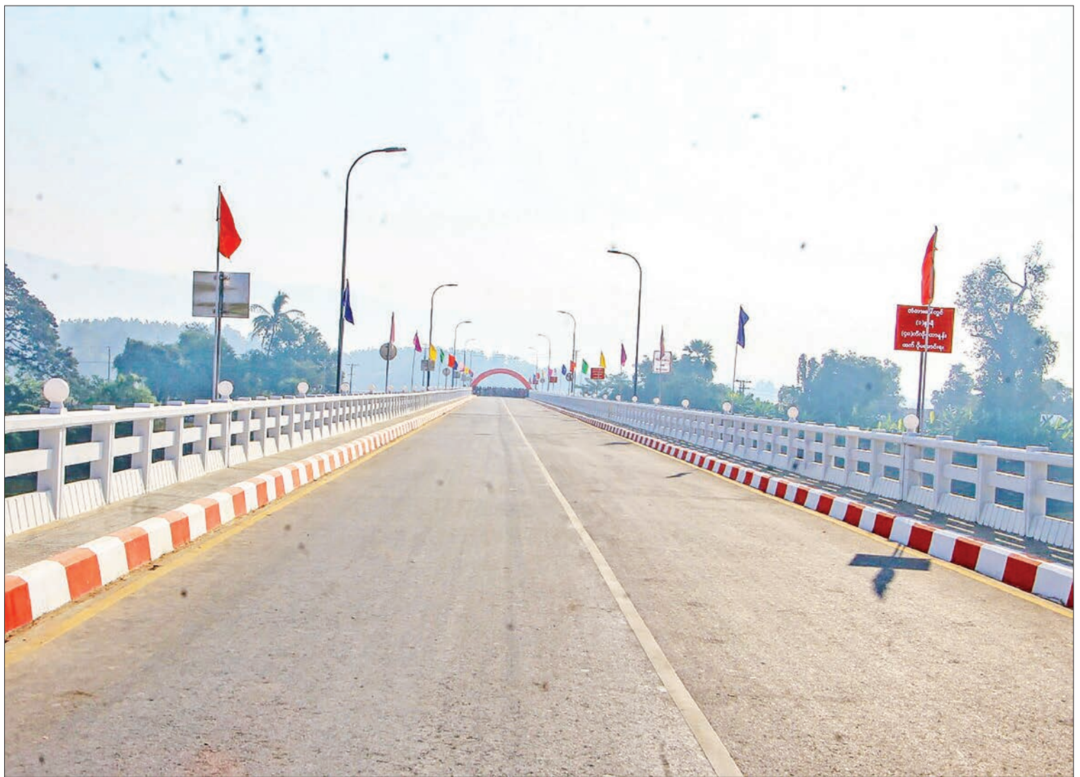
Sittoung River-Crossing Bridge was opened on 2 January 2021 in the commemoration of the 73 rd Independence Day. PHOTO: MNA
