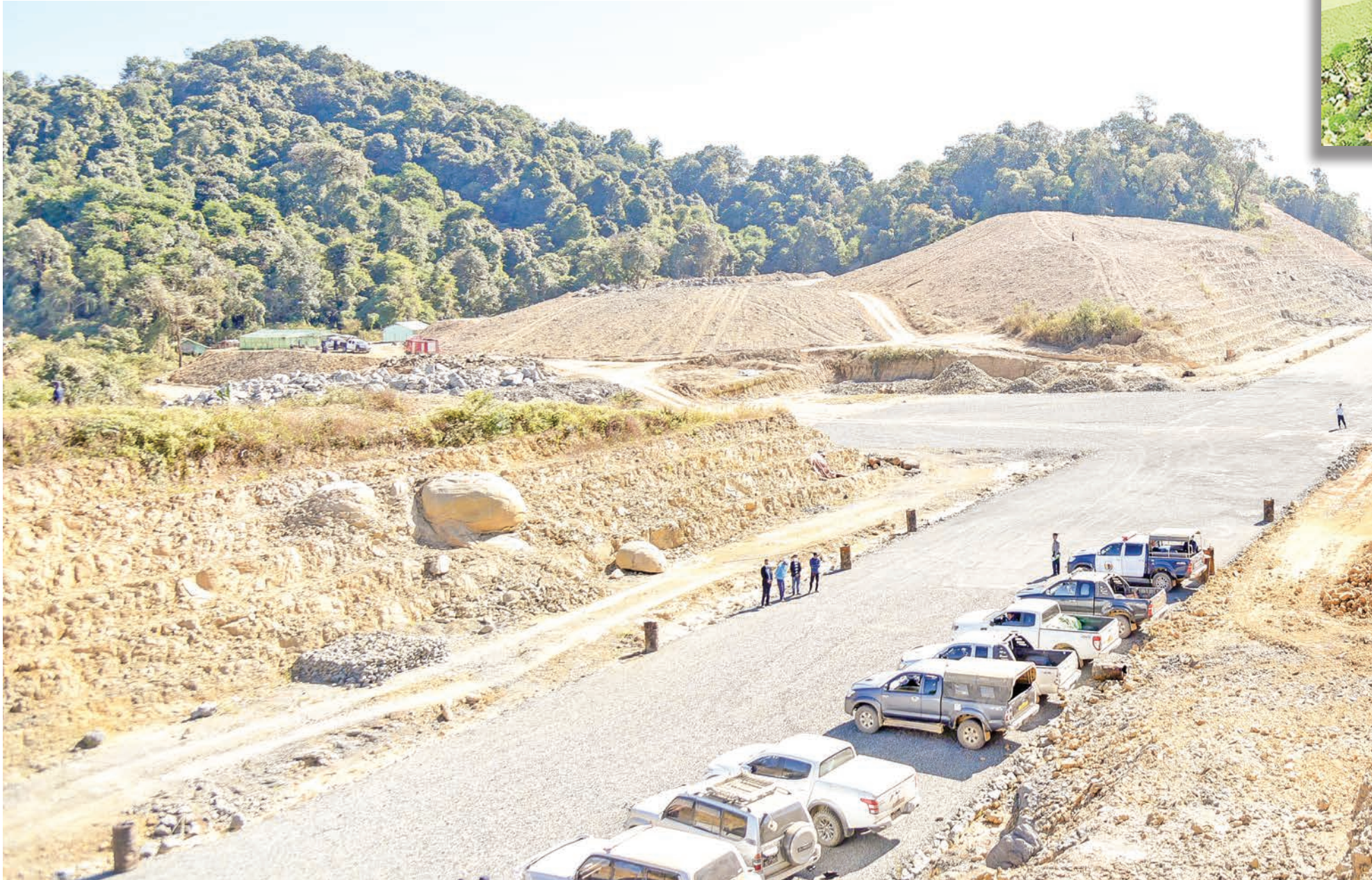
Lailenpi airstrip in Matupi Township is under construction. PHOTO: MNA
