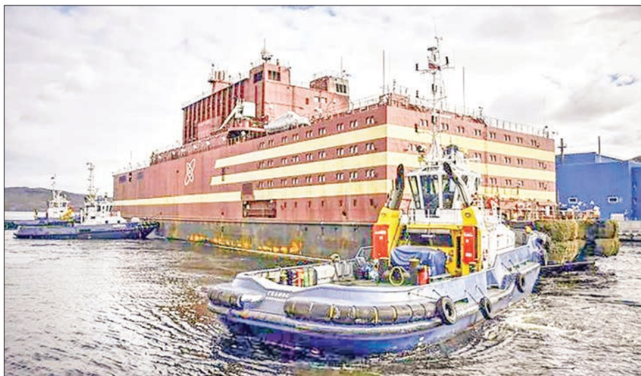
Akademik Lomonosov is a non-self-propelled power barge that operates as the first Russian floating nuclear power station.
