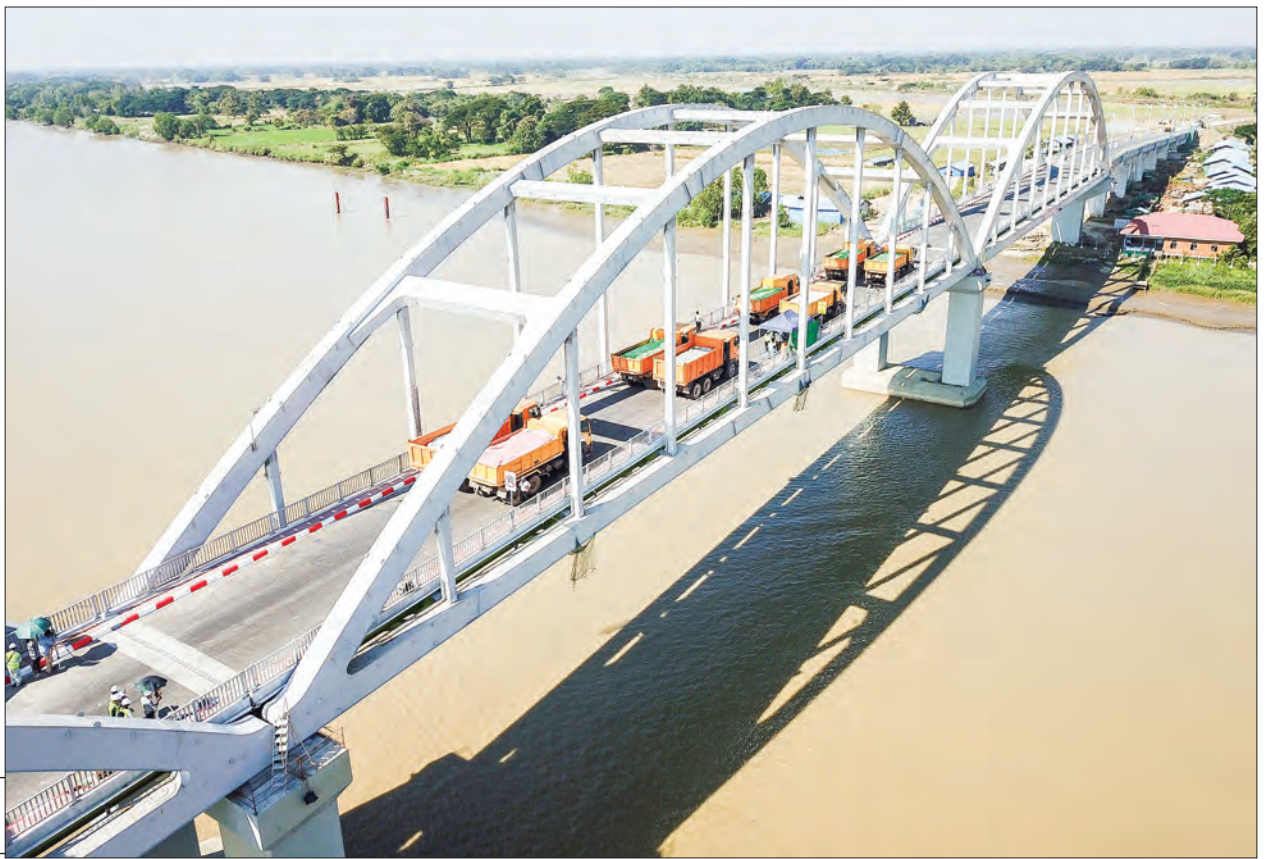
Load testing of the Kyunpyathat Bridge (Tha-yoot-myike) is conducted on 16 December 2020.
