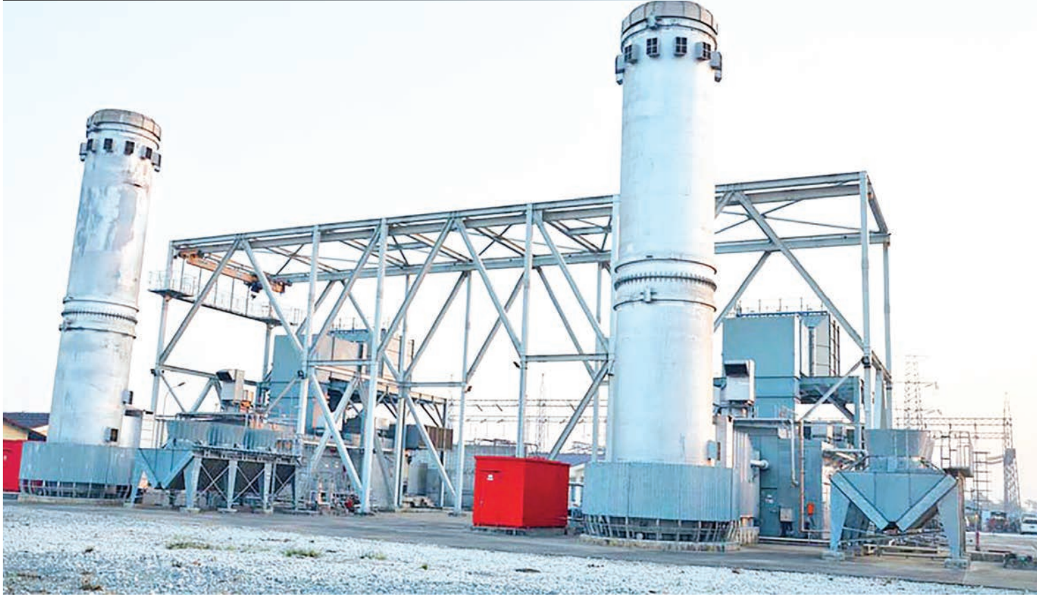
The photo shows a power plant is under construction in Yangon.
