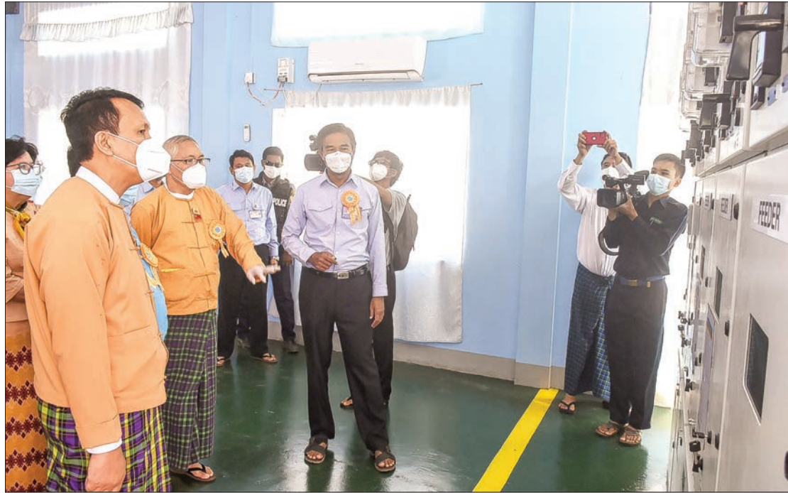
Yangon Region Chief Minister U Phyo Min Thein inaugurates Painkan Power Plant and Zwepalai Power Plant sub-stations in Kayan Township on 27 November 2020. PHOTO: SAN KYAW OO (IPRD)
