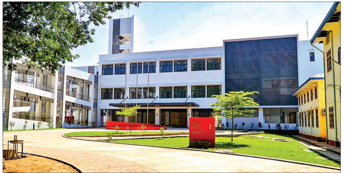
Picture shows the newly-constructed Obstetrics, Gynaecology and Neonatal Ward at the Magway General Hospital in Magway. PHOTO: THAN NAING OO
