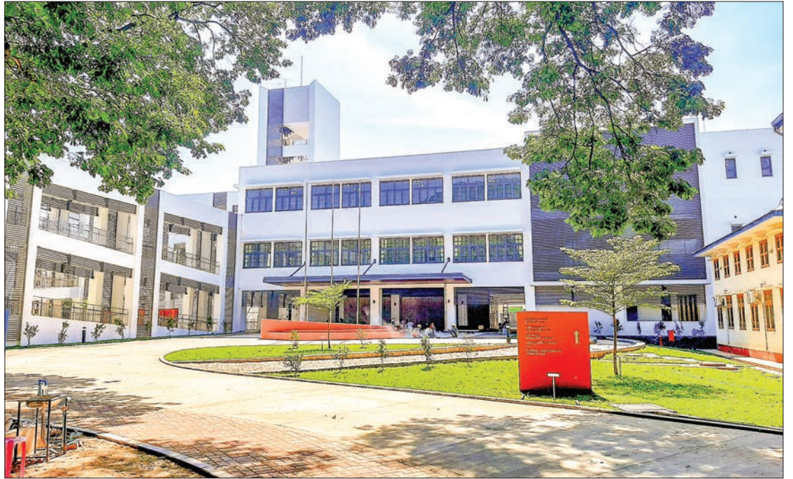
Picture shows upgrading Magway hospital. PHOTO: ZAYYATU(MAGWAY)
