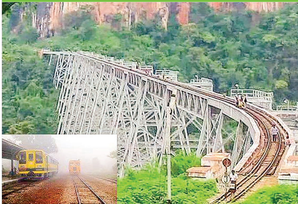
Panorama view of Gokteik Viaduct.
