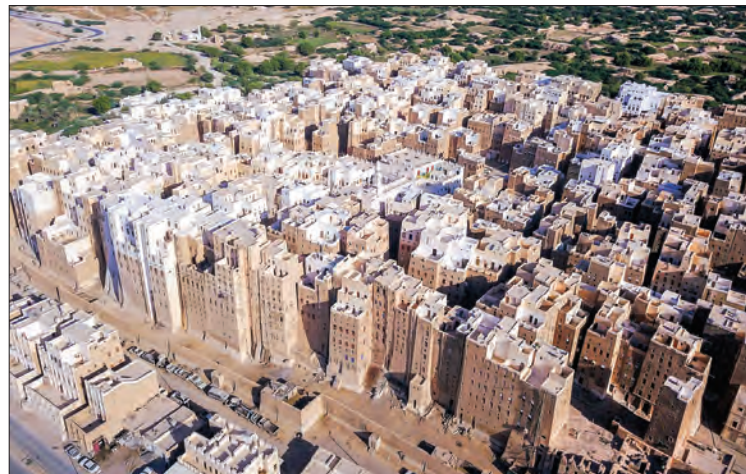
An aerial picture taken on 17 October 2020, shows a view of Shibam City in Yemen's central Hadramawt governorate. PHOTO: AFP
