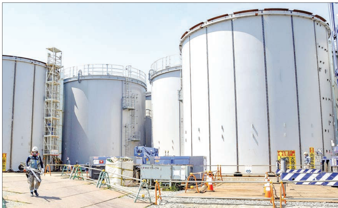
Photo taken Aug. 26, 2020, at the crippled Fukushima Daiichi nuclear power plant in northeastern Japan, shows tanks for storing treated water from which most of the radioactive contamination has been removed. PHOTO: KYODO
