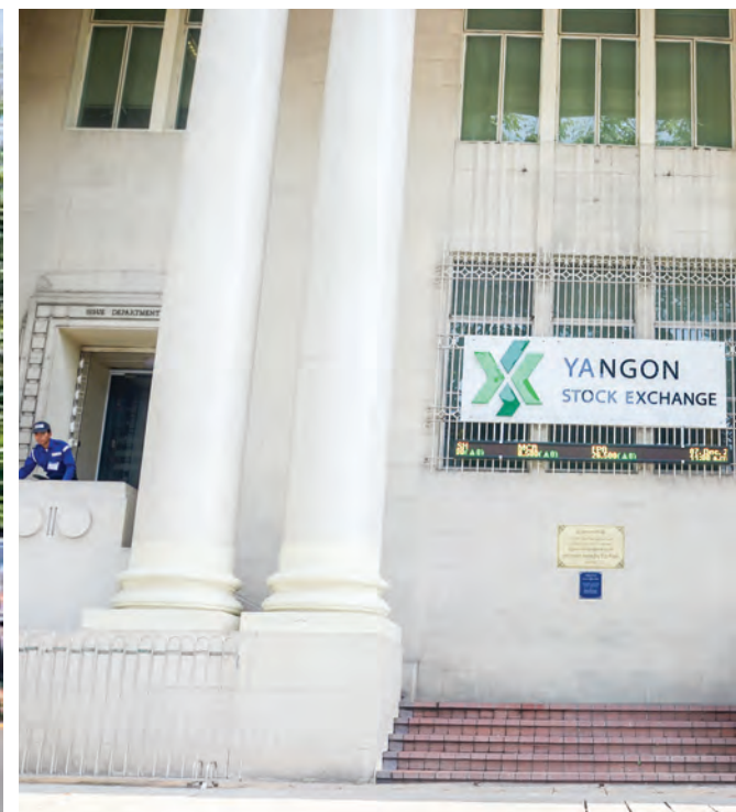
The Yangon Stock Exchange Building in Yangon. PHOTO: PHOE KHWAR
