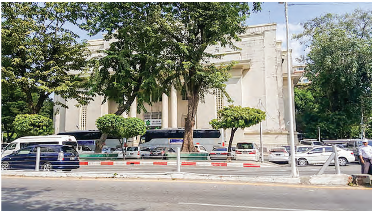
The Yangon Stock Exchange Building in Yangon. PHOTO: PHOE KHWAR
