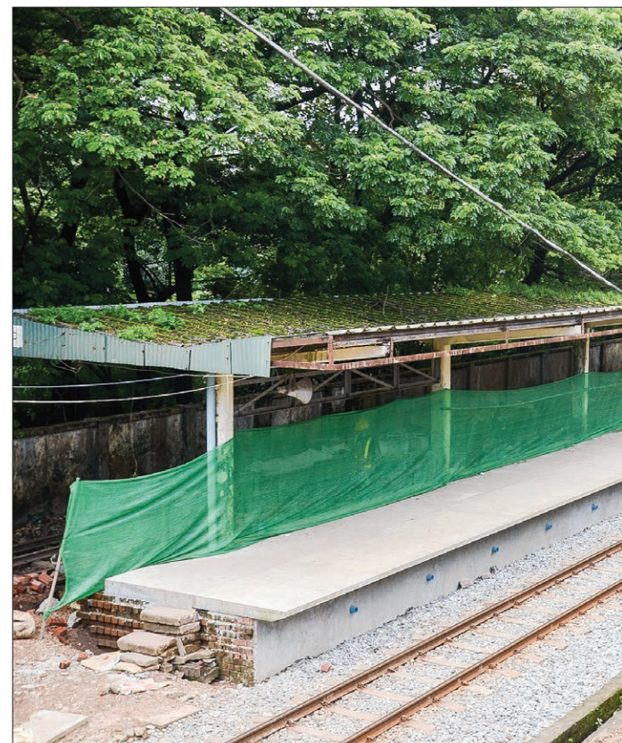
The platform at the Mahlwagon station is begun upgrading. (6459)
