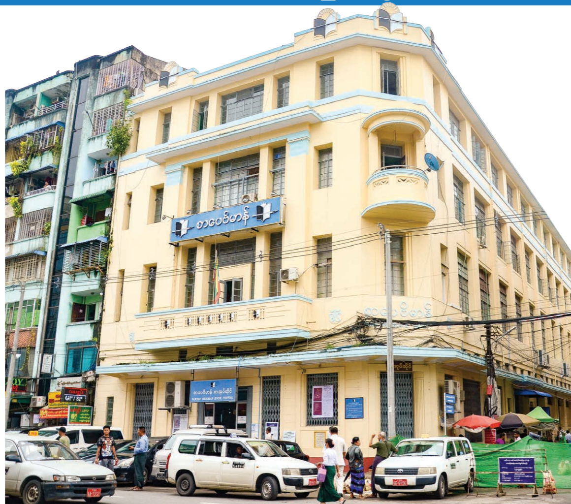
Sarpay Beikman Building in downtown Yangon. PHOTO: PHOE KHWAR
