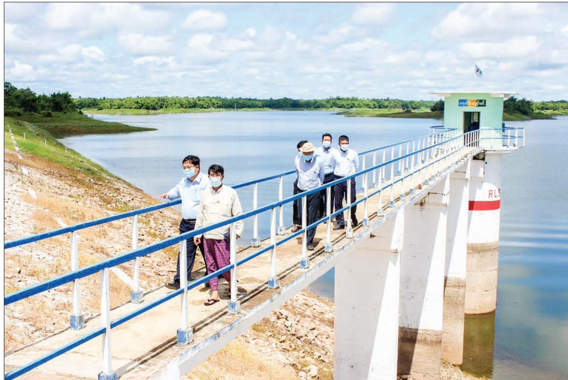
Officials inspect the Chaung Ma Nge Dam in Nay Pyi Taw on 26 July 2020. PHOTO: HTET HLYAN
