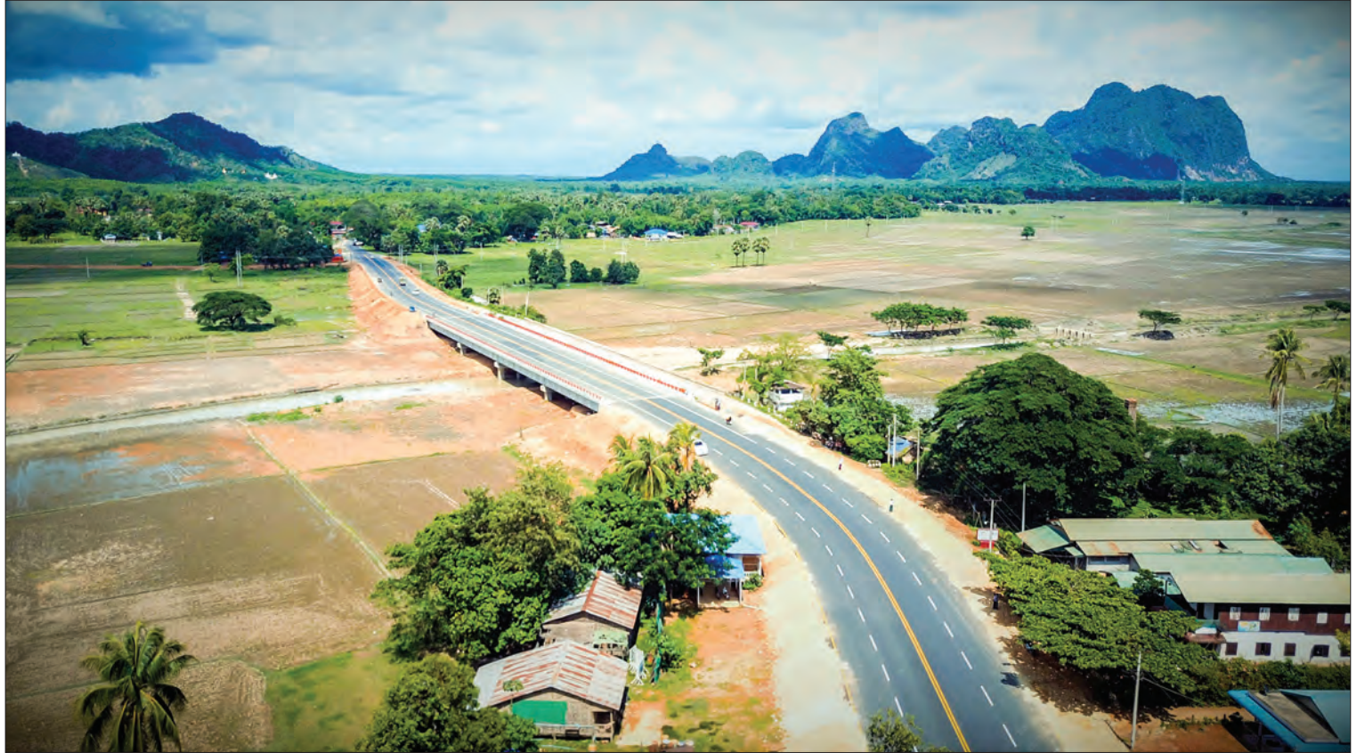
The new Naung Lone Bridge in Hpa-an Township, Kayin State, completed on 5 June 2020 makes better communication for local people. PHOTO: SAW MYO MIN THEIN (IPRD)
