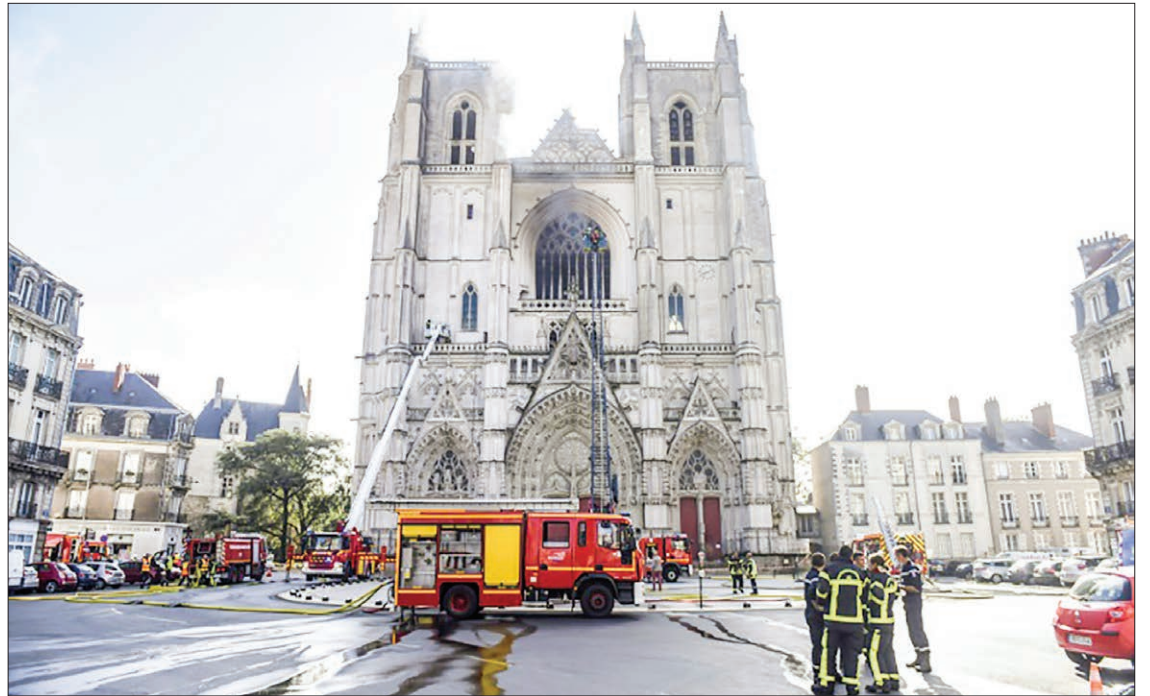
Emergency teams managed to contain the fire at the gothic structure, built between 15 th and 19 th centuries. PHOTO: AFP
