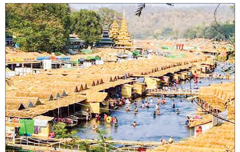
A hotel zone project will be established on the 60-acre land near Shwesettaw pagoda in Minbu district of Magway Region. PHOTO: ZAYYATU (MAGWAY)
