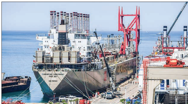
Floating electricity plants known as powerships come into their own when conflicts or other crises make the construction of land-based power stations difficult. PHOTO: AFP
